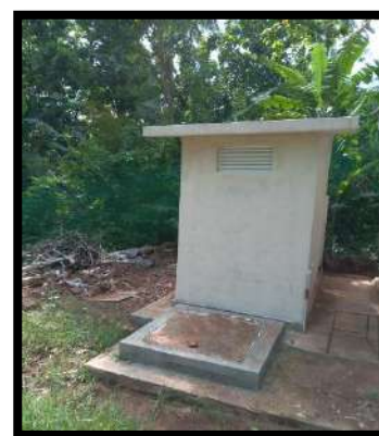
Construction of a single-unit sanitation system at Pelihudugolla K.V. - Completed 100% (LKR 0.82 Million)
