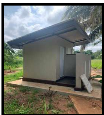
Construction of two-unit sanitation systems at Nikula Bibile K.V. - Completed 100% (LKR 1.14 Million)
