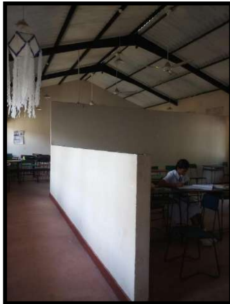
Repair of Two-Story Building at Nalanda M.V.
