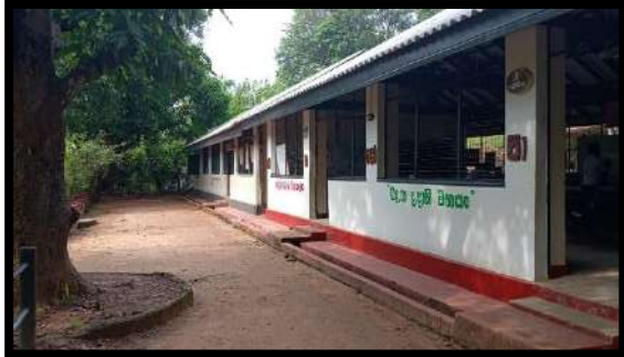
Repair of 80' * 20' Building at Pubbiliya K.V.
