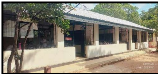
Repair of 60' * 20' Building at Nikula Bibile K.V.
