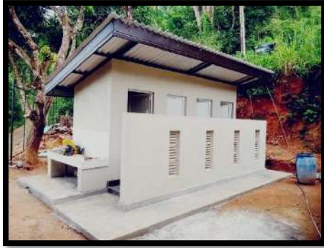
Construction of a four-unit sanitation system at Rattota Mahabodhi K.V. - Completed 100% (LKR 2.5 Million)
